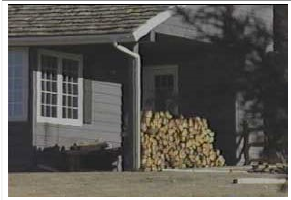
Photograph 12.3. Improper Placement of Firewood
