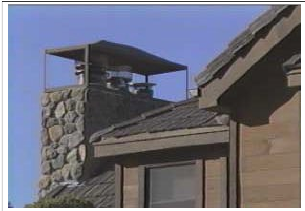
Photograph 11.2. Chimney/Stovepipes with Spark Arresters
