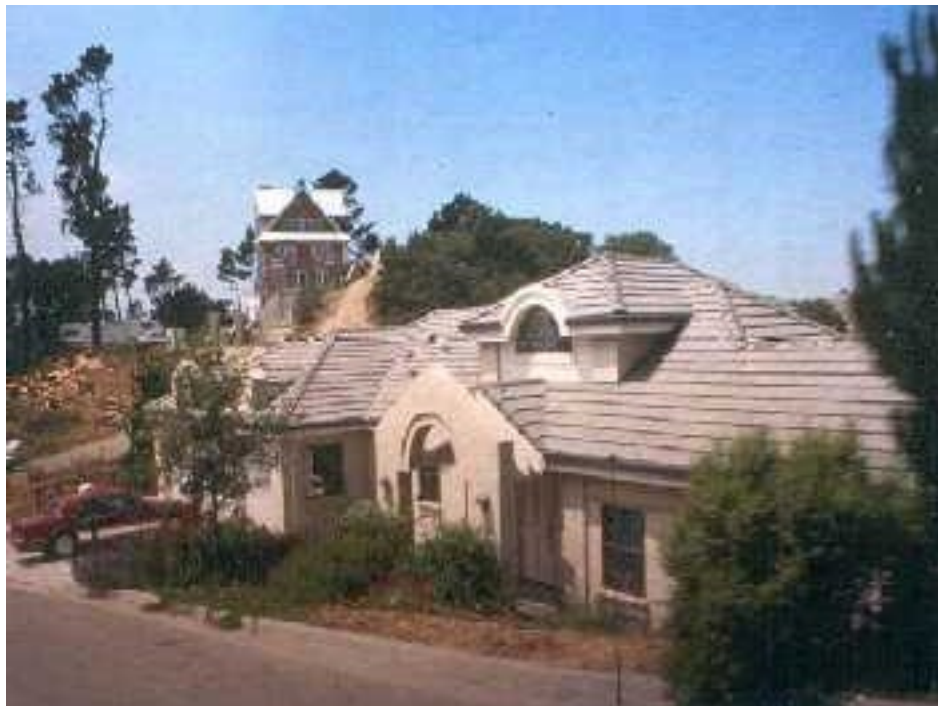
Photograph 11.1. A Clean, Well-Maintained Class A Roof
