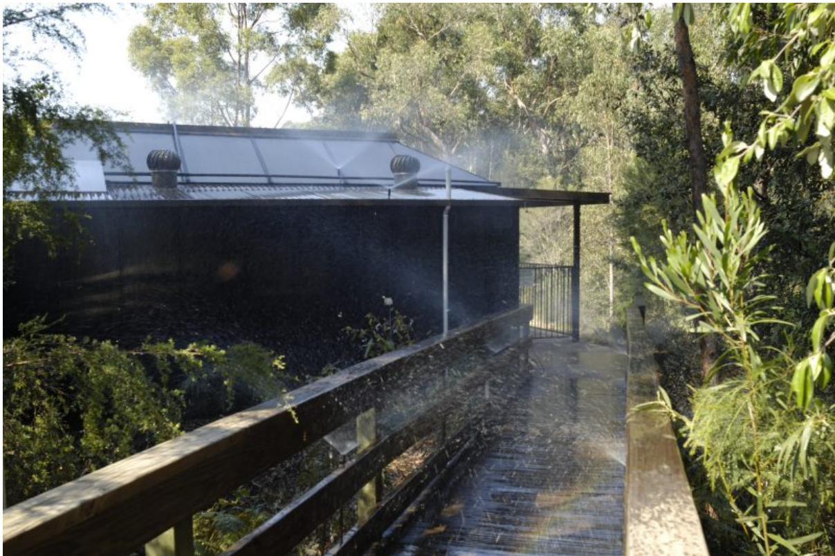
Figure 7. External Sprinklers. As a wildfire approaches, external sprinklers wet the structure at risk, the surrounding environment, and increase the local humidity to prevent ignition. Photo: A conference center in New South Wales, Australia.
